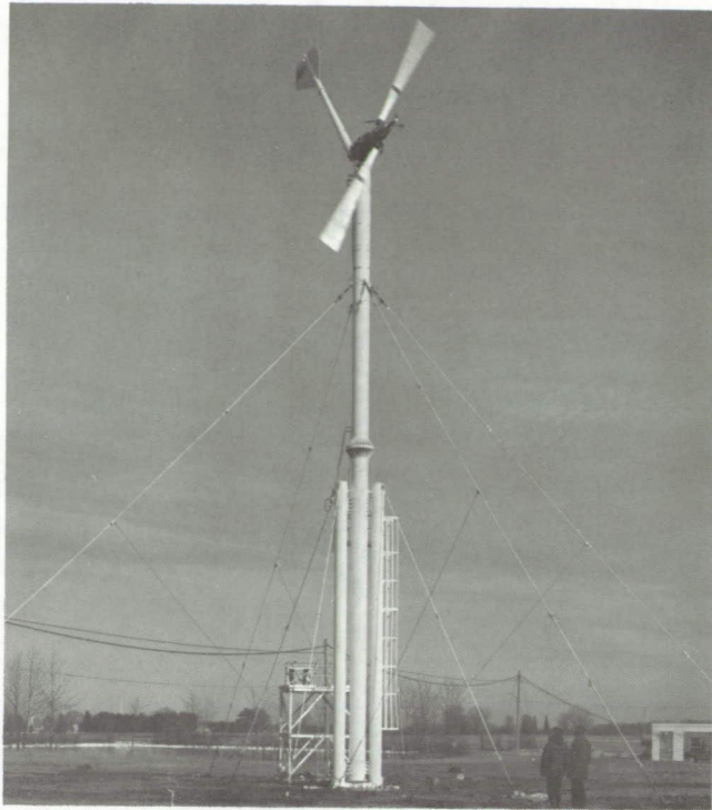
Figure XI-27. - Four-kilowatt wind turbine generator.
